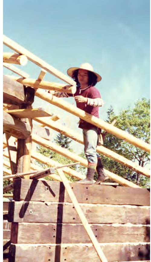
Constructing the roof, 1976.
