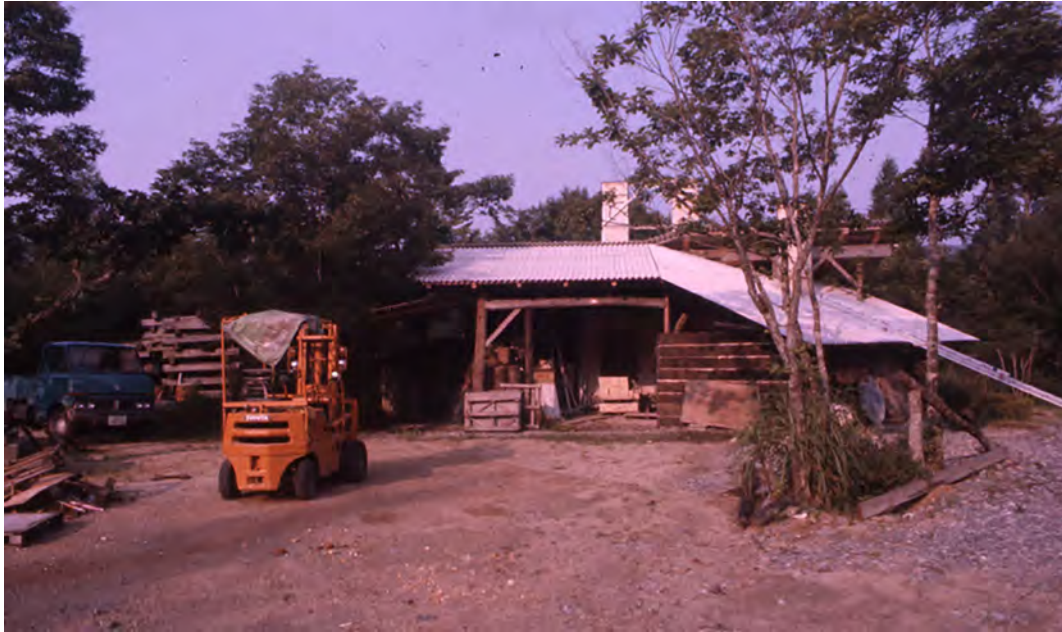
Kaneko's completed studio in Nagura, Japan, 1978.
